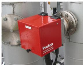
The heated probe contains a heated ceramic filter of suitable pour size to filter out carbon dust from the beds.
